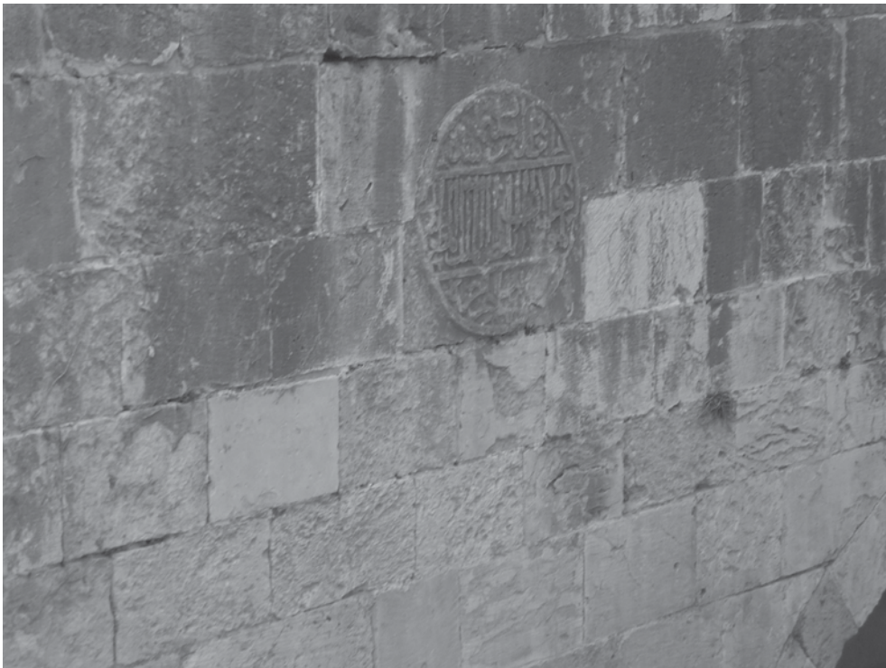
Fig. 6 inscription 5 Stone bridge Citadel entrance
